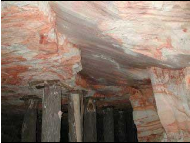
Fault plane (smooth surface) exposed in the sandstone roof of an opal mine, Coocoran opal fields, Lightning Ridge.
