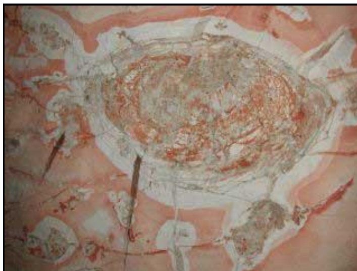
Blow (light coloured circular area) about 1.2 metres across exposed in the sandstone roof of a mine, Coocoran opal fields, Lightning Ridge.
