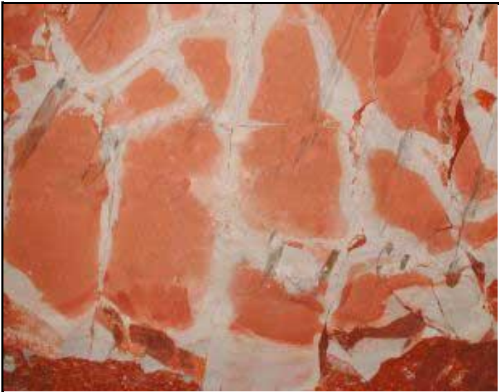
Joints (light coloured) exposed in the sandstone roof of a mine, 3 Mile opal field, Lightning Ridge.
