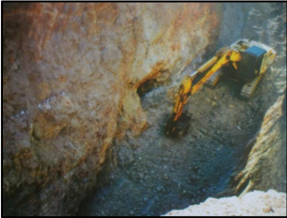
Open cut over the old working.
